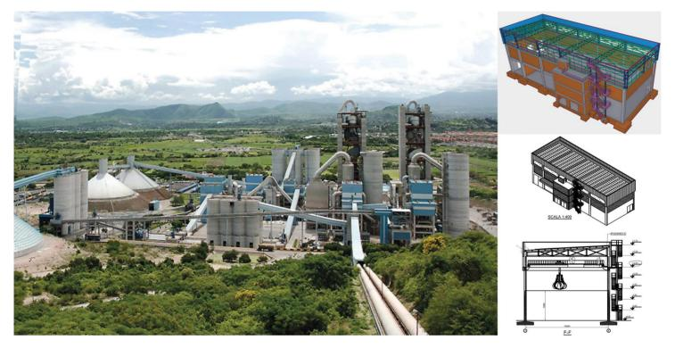
Construction project of a storage building for alternative fuels for the Tepetzingo cement plant (Mexico) with plan dimensions of 52.7x20m and an approximate height of 19.6m. The structure is made of concrete frames up to the support level of the bridge crane and steel roof with maximum distances between frames of 11.75m. Warehouse detailed design, including workshop documentation and detailing
